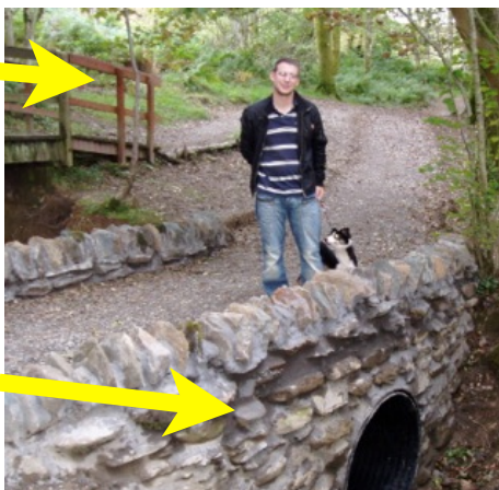
The new culvert-bridge.
